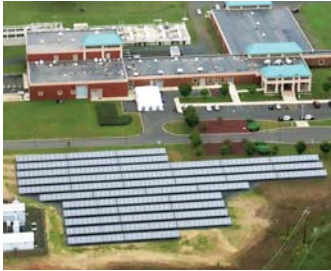
Canal Road Treatment Plant in Franklin, NJ.
