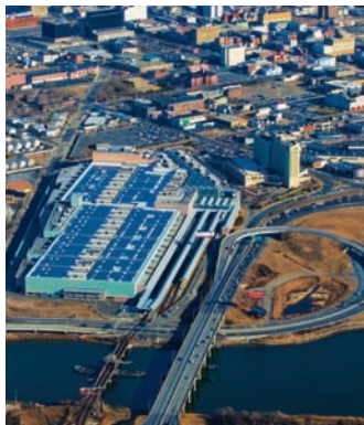
The ACCVA installed a 2.37 MW solar system in 2008.
