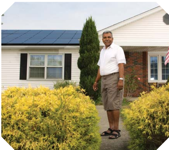
Ralph Byrd, of Egg Harbor Township, reduced his carbon footprint by installing solar panels, which eliminated 13,230 pounds of carbon dioxide from the air. That is the equivalent of removing one car from the road for one year.
