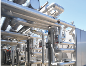
Viking technicians devised this elaborate piping for the absorption chiller, which produces plant cooling for the company's tri-generation system.
