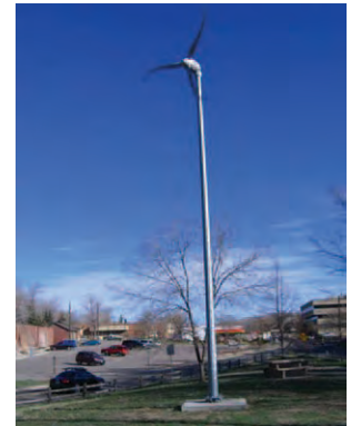
Skystream 1.8kW turbine
