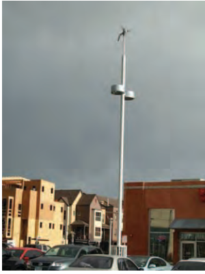
Southwest Windpower "Air" on lamppost
