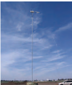
Guyed Monopole Tower
