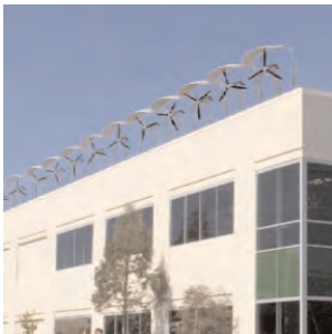
AeroVironment rooftop array
