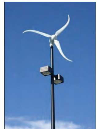
Skystream 1.8kW turbine dual-use on lamppost
