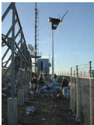
Proven Energy 6kW turbine powering telecommunications equipment
