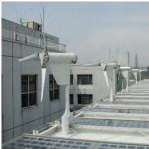
Proven Energy 2.5kW turbine rooftop array
