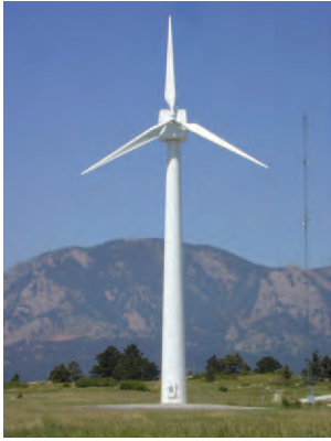
Northern Power 100kW turbine
