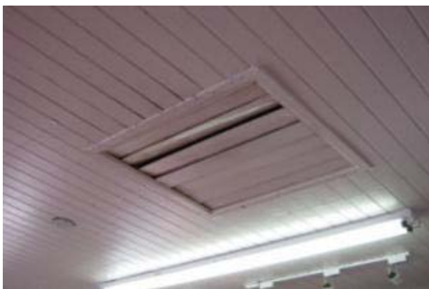
Louver opens to roof Belmar Borough- Taylor Pavilion
