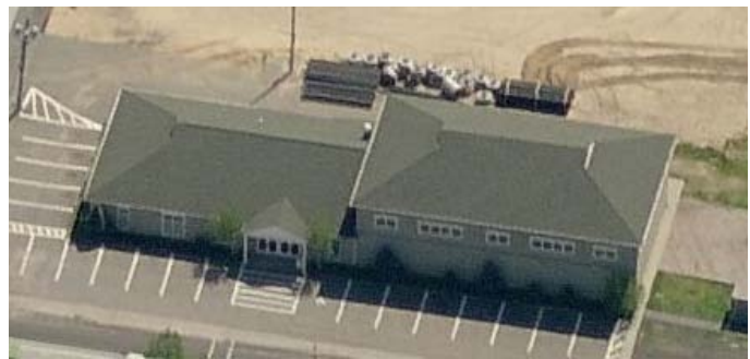
Aerial view of roof, Bing Maps
