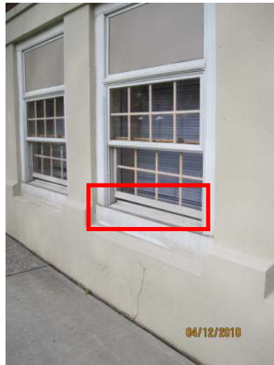
Window not closing all the way, warped
