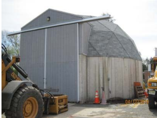
Front Façade Salt Dome
