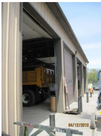
Front Façade Steel Garage
