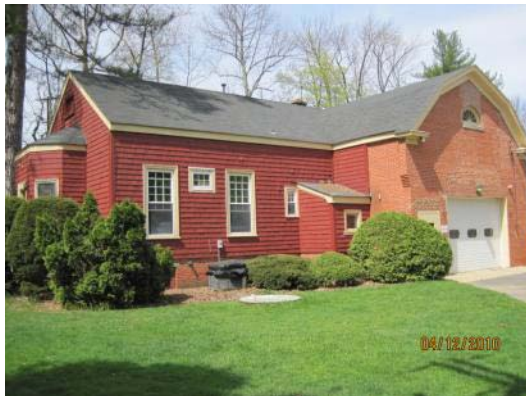
Front and Side Façade
