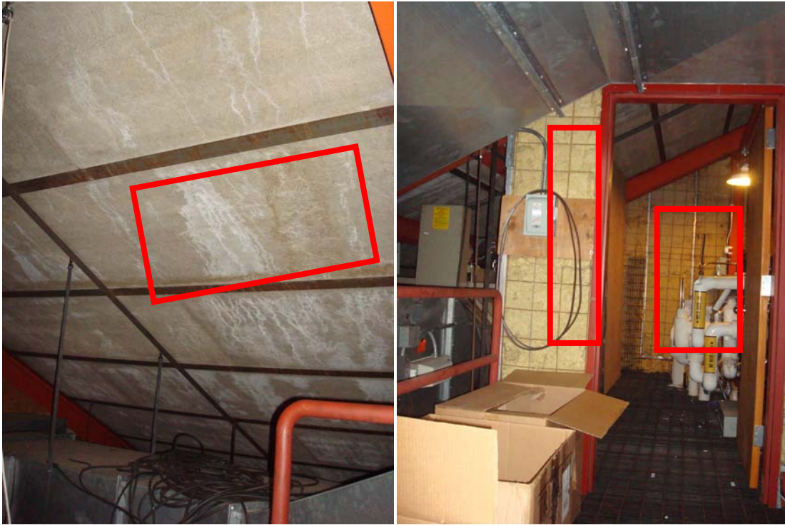
Fiberglass boards/planks supporting slate roof; attic wall Rockwool insulation
