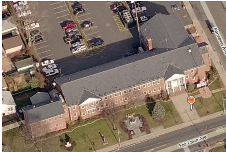
Bird's Eye View of Building, roof dark spots indicate damaged/missing tiles
