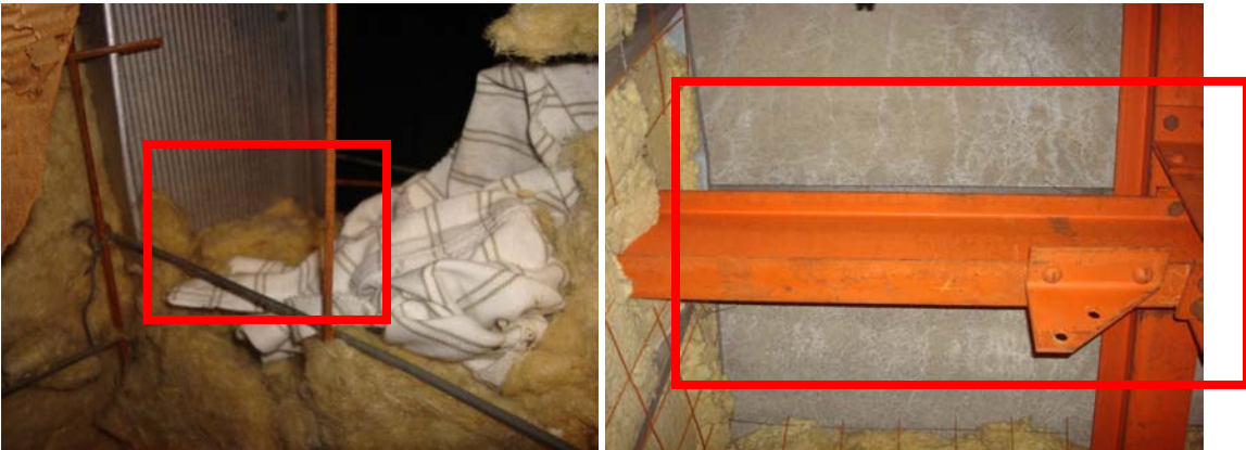
Attic outer wall 8" Rockwool insulation; steel trusses supporting slate roof
