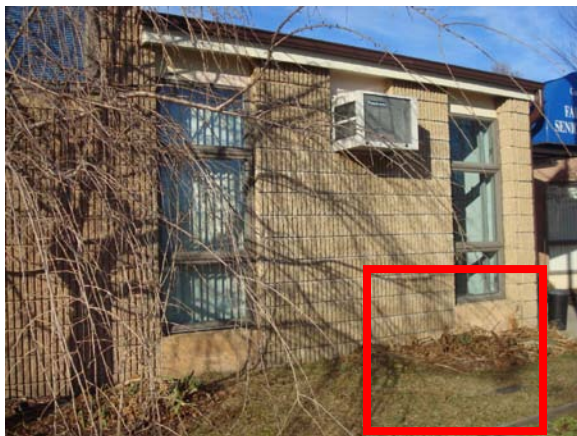
Exterior wall ribbed and stucco
