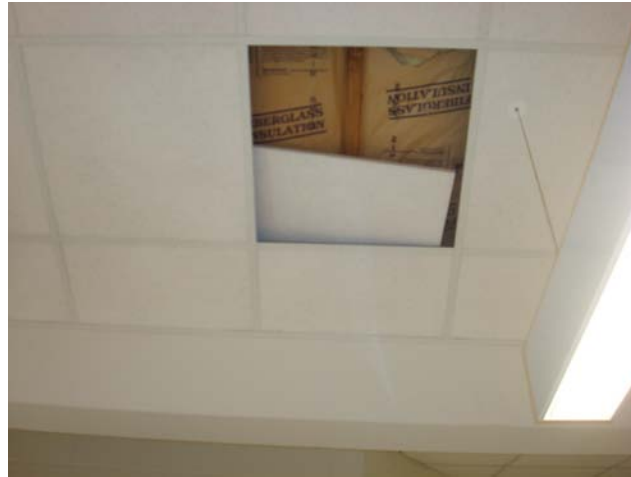
R-19 batt insulation in-between drop ceiling and roof support
