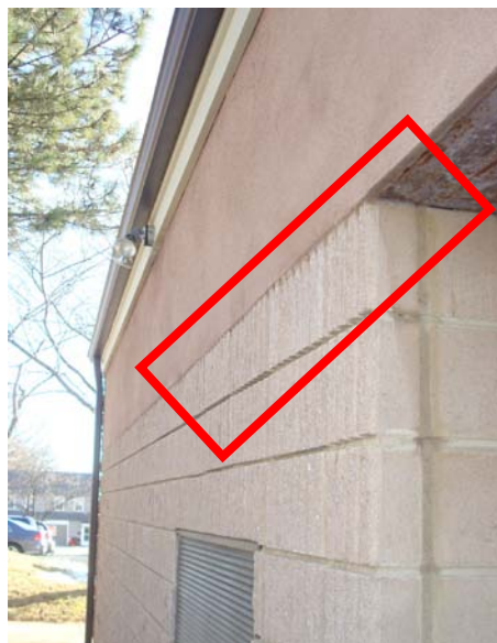
Exterior wall ribbed and stucco
