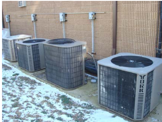
York condensing units located outside
