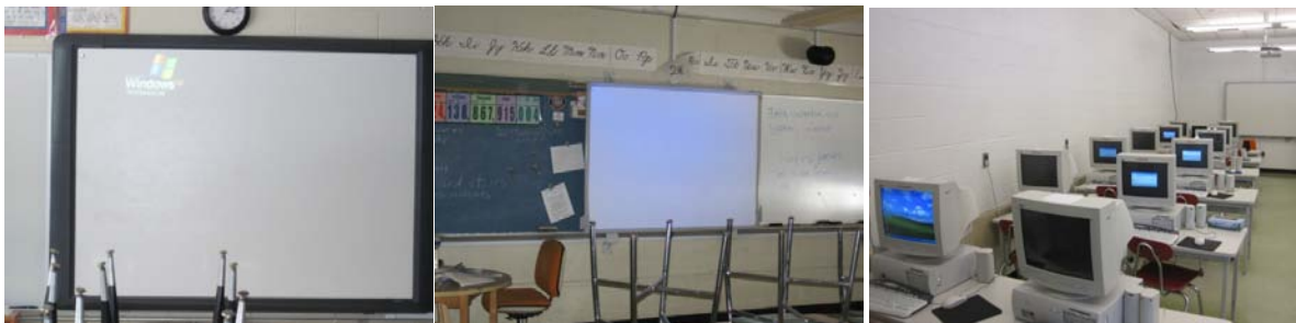
Smartboards & Computers left on in vacant classrooms
