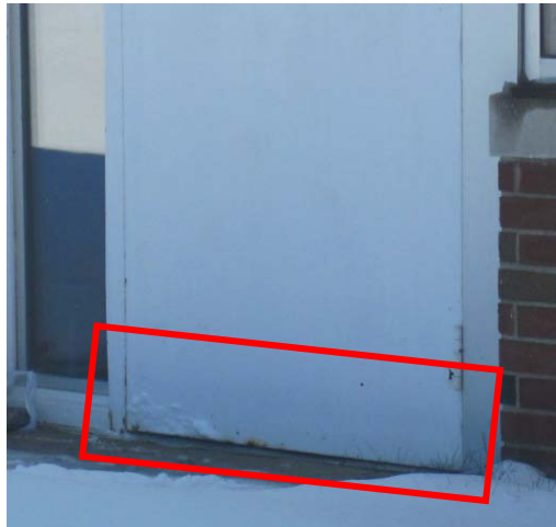
Older exterior wood door (serving as exit from classroom)
