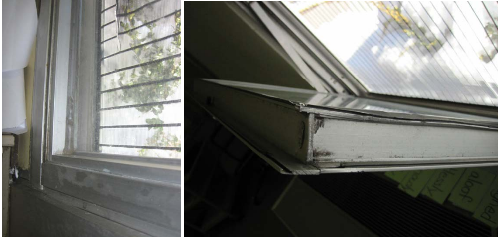
Single pane aluminum framed windows
