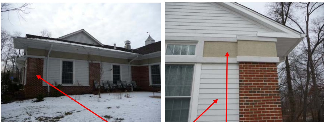
Façade brick veneer, HardiPlank and stucco finishes
