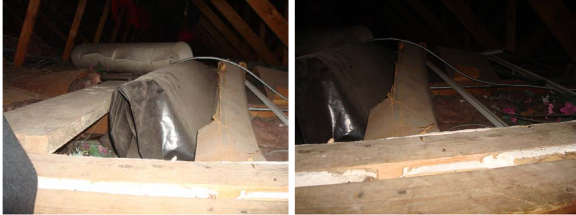
Insulation in the mezzanine floor area
