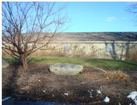
DPW back side continuous asphalt shingle earth colored roof
