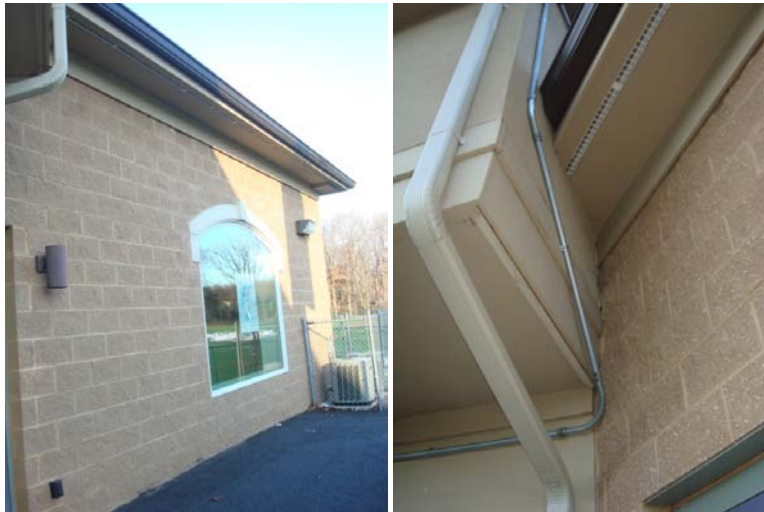
Façade: split face concrete blocks, EIFS (second floor), and cinder blocks (below)
