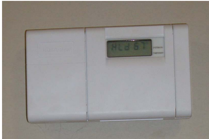
Attic programmable thermostat, set at 67°F at all times
