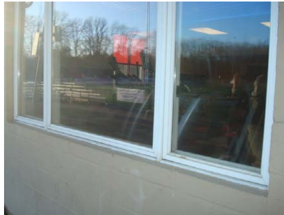
First floor windows
