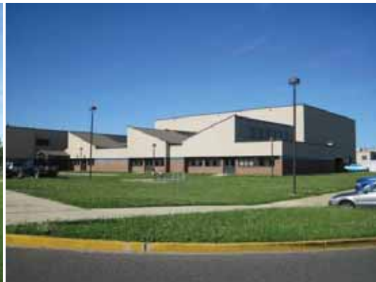
Partial Rear Façade (typ.)
