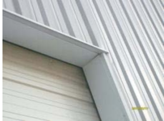
Door does not close with an air tight seal and is missing weather stripping
