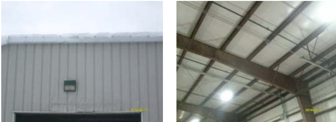
Typical roof and view of the steel structure from the interior
