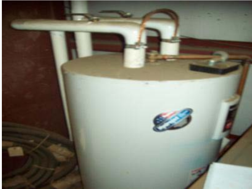
Bradford-White electric domestic hot water heater
