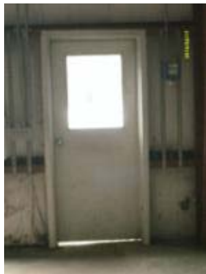
Door does not close with an air tight seal and is missing weather stripping
