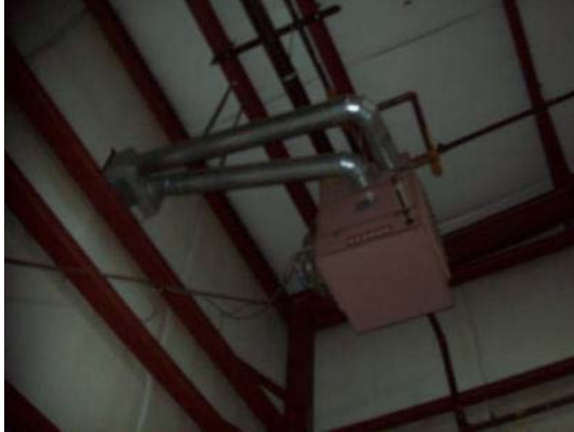
Reznor gas-fired convective heating unit
