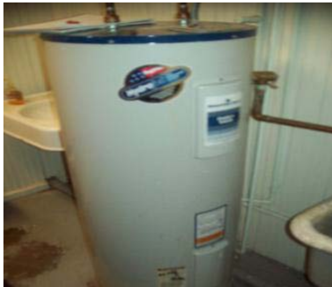
Bradford-White electric DHW heater
