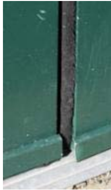
Doors not closing completely and missing weather stripping
