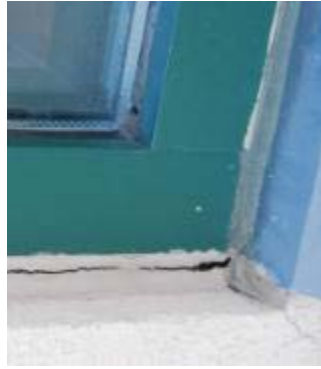
Cracked caulking at windows
