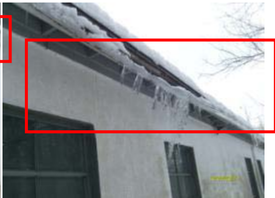
Examples of damaged fiberglass insulation, and damaged roof drainage around gutters.
