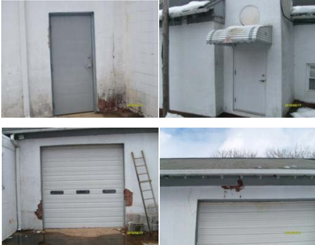
Typical exterior doors that are in good age appropriate condition
