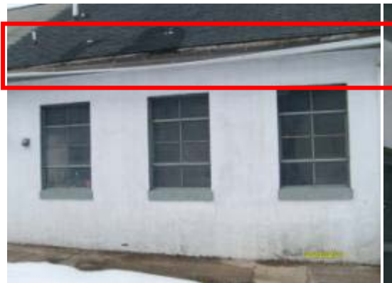
Examples of damaged fiberglass insulation, and damaged roof drainage around gutters.
