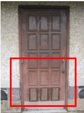
Warped and aged door and frame
