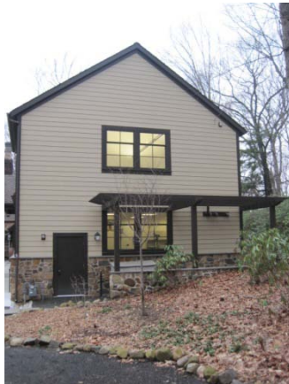
Partial Right Side Façade (typ.)
