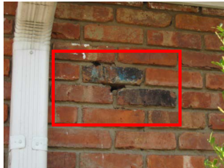
Exterior wall penetrations in brick facade
