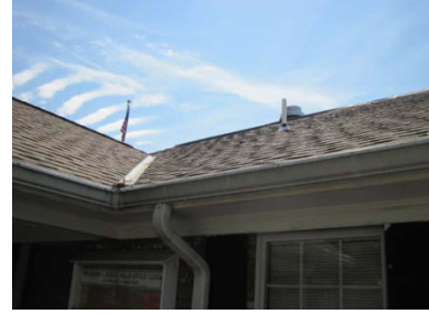
Asphalt shingle roof in good condition
