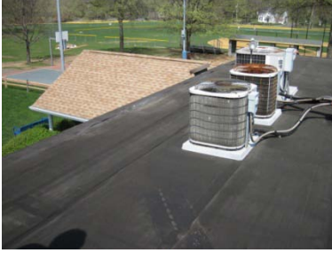
EPDM roof membrane in good condition
