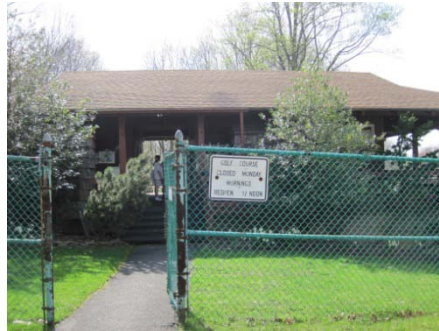
Asphalt shingle roof in good condition
