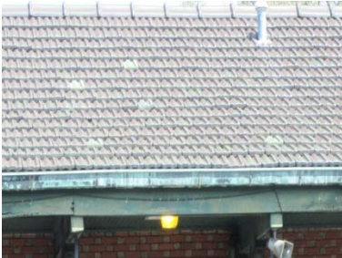
Ceramic tile roof in good condition
