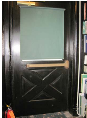
Exterior door acceptable condition
