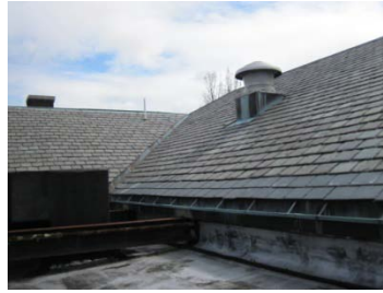
Typical slate shingle roof image
