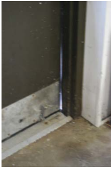
Missing/worn weatherstripping
