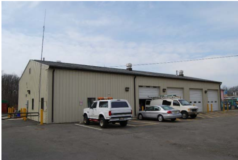
Front and Left Side Façade
