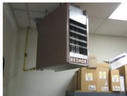
Gas-fired Furnace in office & Unit Heater in Sign Room.
