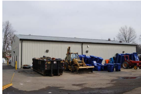
Rear and Right Side Façade
