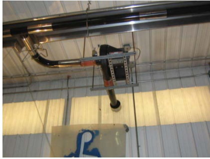
Infrared heating system vacuum pump (left) and tube section
