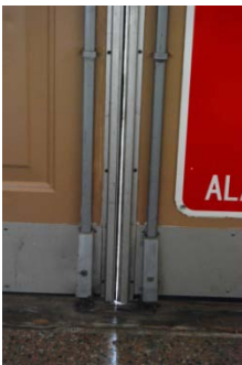
Missing/worn weather-stripping
