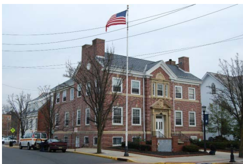
Front and Left Side Façade
