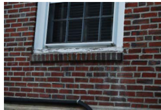
Cracked/deteriorated bricks and mortar joints due to water infiltration through window sills and chimney flashing.
