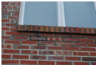
Cracked/deteriorated bricks and mortar joints due to water infiltration through window sills and chimney flashing.
