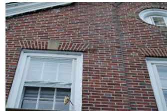
Cracked/deteriorated bricks and mortar joints due to water infiltration through window sills and chimney flashing.
