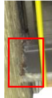
Substantial structural damage visible on interior structural members caused by water inside the envelope assembly
