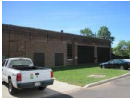
Partial Front Façade
