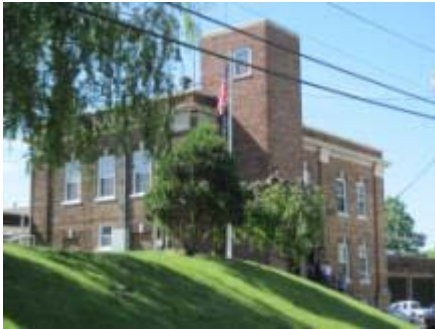
Front and Left Side Façade
