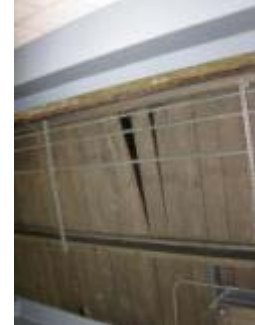
Water damaged ceiling tiles and wood paneling visible in the interior
