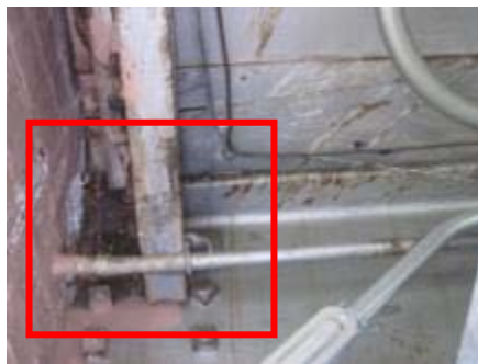
Substantial structural damage visible on interior structural members caused by water inside the envelope assembly
