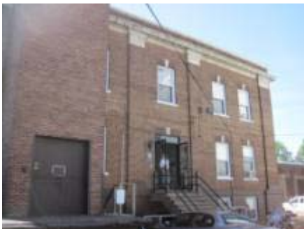
Partial Front Façade
