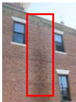
Missing downspouts leave signs of water damage on façade.
