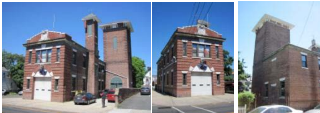
Front and Right Side Façade
