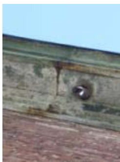
Missing downspouts leave signs of water damage on façade.
