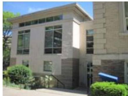
Partial Left Side Façade (typ.)
