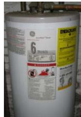
Figure 3: 30 gallon GE water heater
