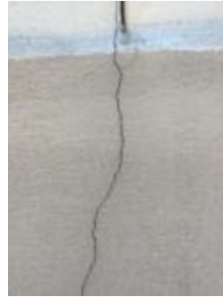
Cracked/deteriorating EIFS/stucco showing signs of water or moisture damage
