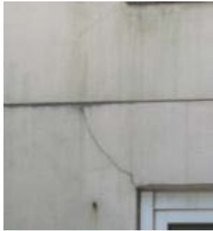
Cracked/deteriorating EIFS/stucco showing signs of water or moisture damage
