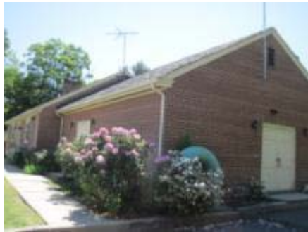
Front and Side Façade
