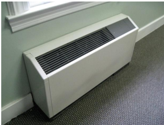
Typical Water Source Heat Pump
