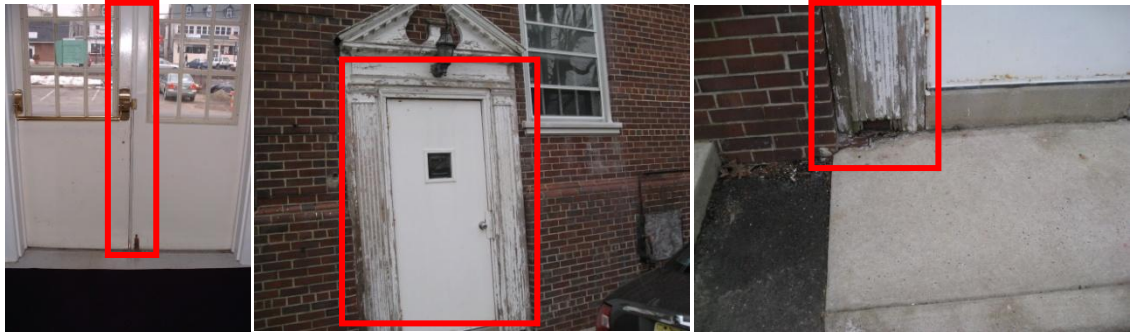
Doors with missing/worn weather stripping; other wood doors with rotting frames
