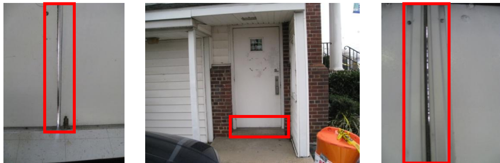
Doors with missing/worn weather stripping; other wood doors with rotting frames
