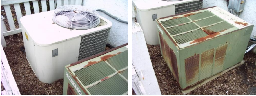
Split System Condensing Units on Grade for Bar and Second Floor Recreation Room
