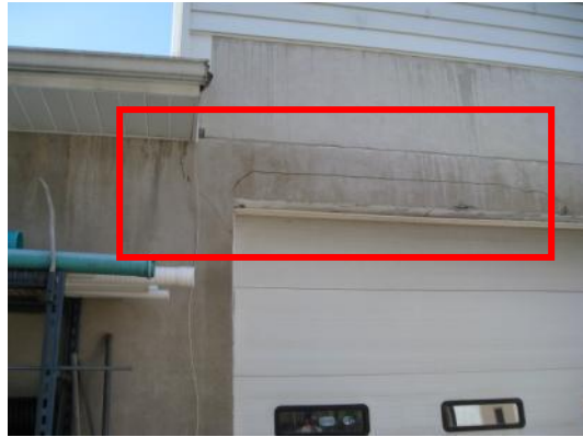
Potential structural damage visible on exterior walls caused by water/ice build-up inside the envelope assembly or building settling
