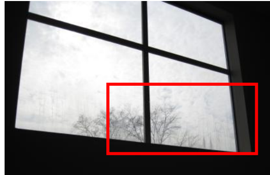
Water damage within window air gap on second floor fixed window
