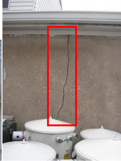
Potential structural damage visible on exterior walls caused by water/ice build-up inside the envelope assembly or building settling
