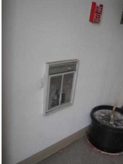
Lobby electric unit heater (left); second floor office AC unit (right)
