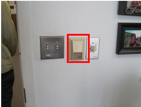
Temperature sensor (middle device - typical)
