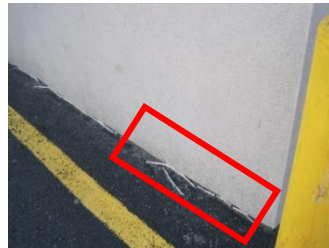
Missing/ineffectively-applied caulk
