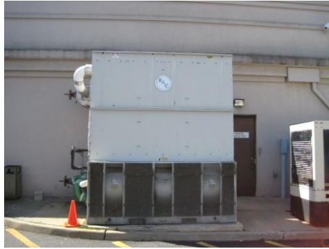
Cooling Tower and water leaking to ground from its corroded basin
