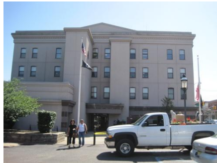
West Façade and Main Entrance
