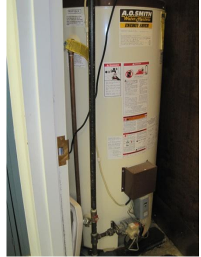
DHW heaters - One electric per floor (left); Under sink electric type (middle); Gas fired unit serving the locker rooms and showers (right)
