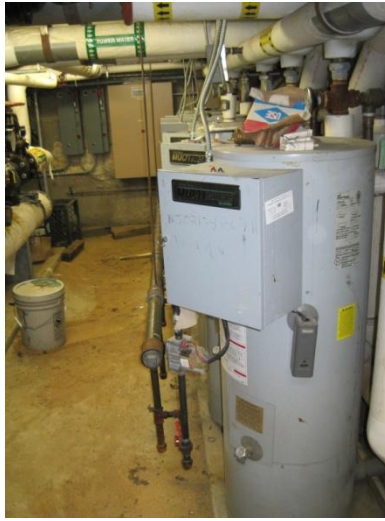
The six Hydrotherm condensing boilers in the boiler room
