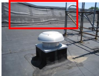
Membrane delamination
