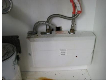
DHW heaters - One electric per floor (left); Under sink electric type (middle); Gas fired unit serving the locker rooms and showers (right)
