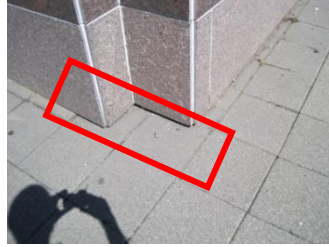
Missing/ineffectively-applied caulk
