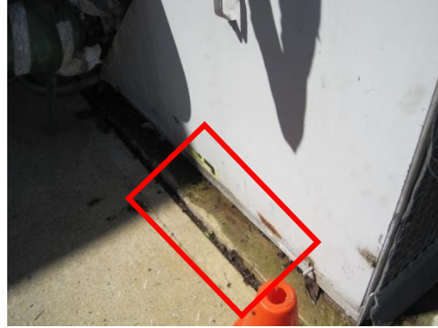
Cooling Tower and water leaking to ground from its corroded basin
