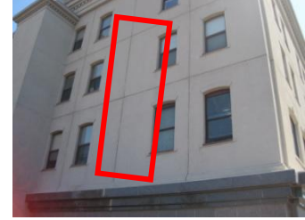
Missing/ineffectively-applied caulk
