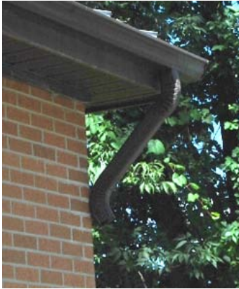
Missing downspout
