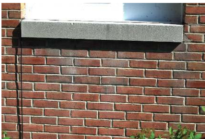
Slightly aged sill caulk and brick veneer Unsealed book drop box sleeve
