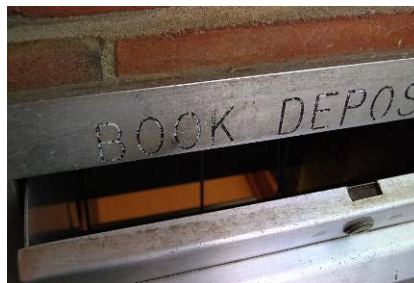
Slightly aged sill caulk and brick veneer Unsealed book drop box sleeve
