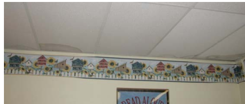
Water damage visible on ceiling tiles in basement perimeter
