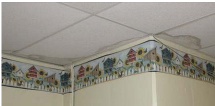
Water damage visible on ceiling tiles in basement perimeter
