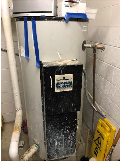
Electric DHW Heater
