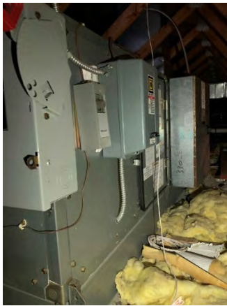
Heating Unit in Attic
