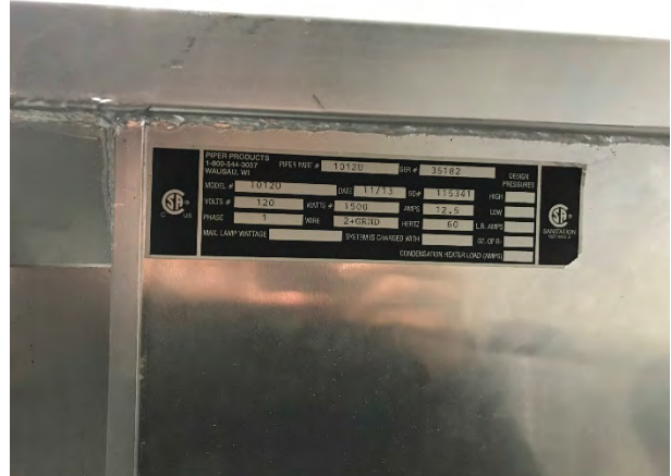
Heated Cabinet Nameplate
