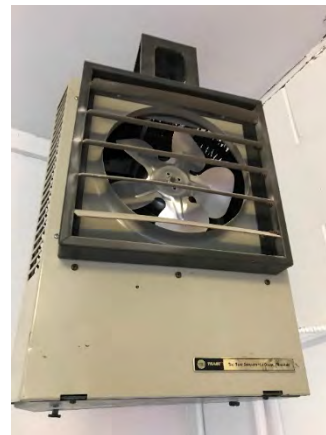
Electric Unit Heater
