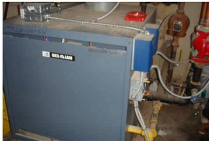
Picture: Old Cast Iron Sectional Boiler Firehouse
