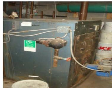
Picture: Library Cast Iron Sectional Boiler
