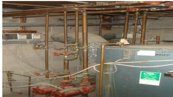
Picture: Firehouse un-insulated pipes
