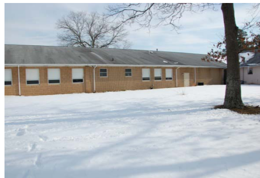
Rear Wing C Façade
