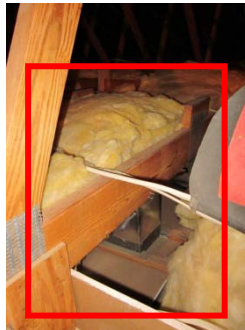
Uneven/ineffective attic insulation found
