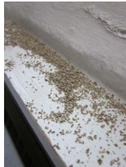
Cement block deterioration and/or insect nesting around interior window cavities
