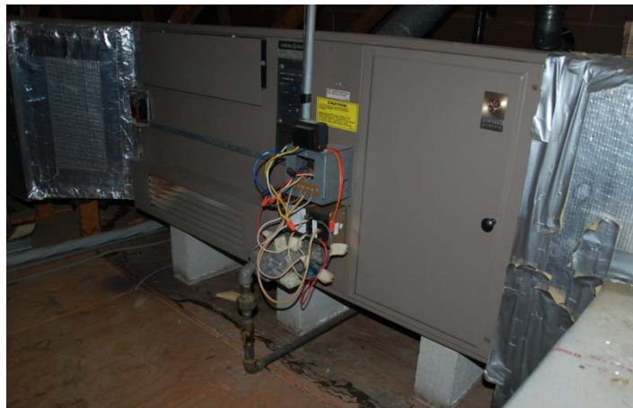
B wing GE furnace
