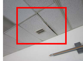
Sagging acoustic ceiling tiles in several areas
