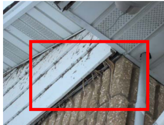
Uncontrolled vegetation growth on roof
