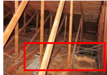
Uneven/ineffective attic insulation found
