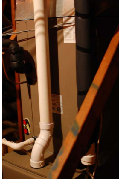
A wing condensing furnace
