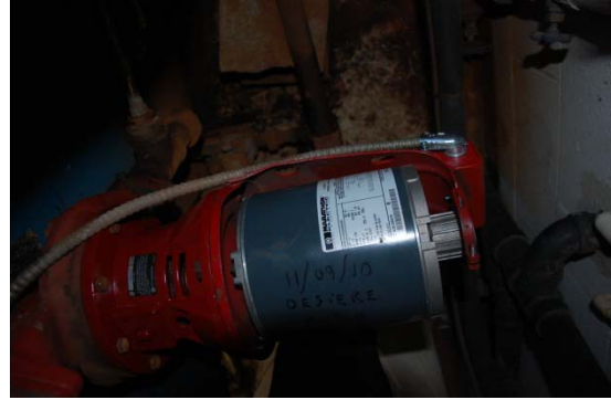
C wing HW Pump
