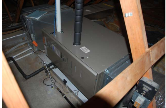
B wing Carrier furnace
