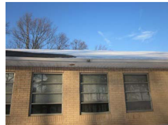
Single-glazed window with ineffective frame
