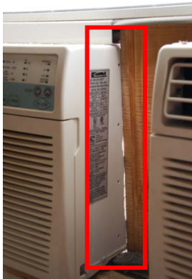
Air-leakage at sleeved wall air-conditioning units
