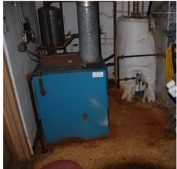
C wing boiler - Columbia
