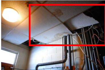
Signs of water damage on ceiling tiles
