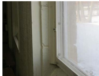
Uninsulated aluminum window frame
