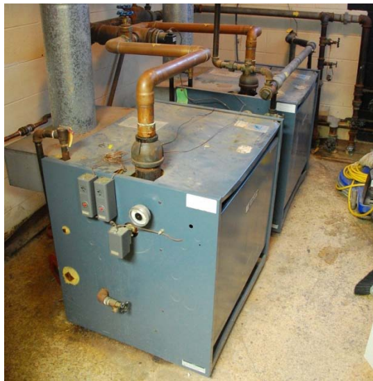
A wing boilers - Weil McLain
