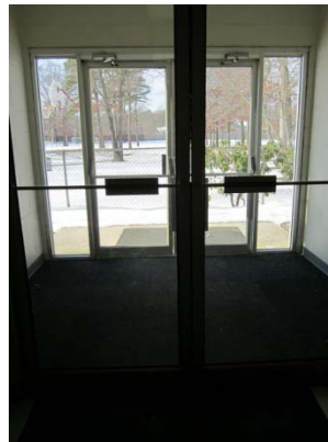
Single-pane glass, uninsulated frame
