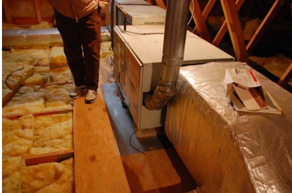
Heating/Cooling furnace
