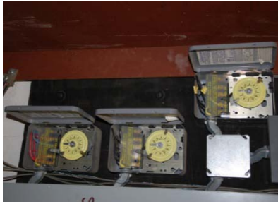
Boilers controls, EMCS and time clocks
