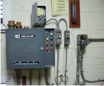
Boilers controls, EMCS and time clocks
