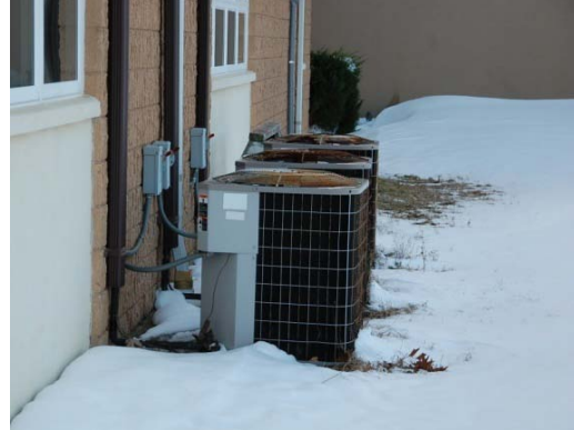
Condensing units outside
