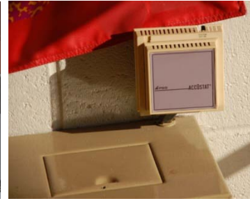
Cabinet heaters and thermostats
