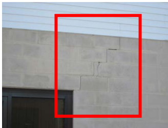
Cracked/deteriorated mortar joints
