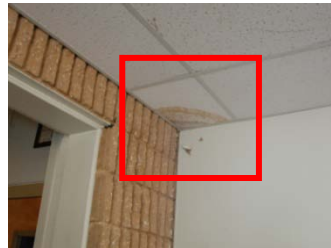
Signs of water damage on interior finishes – Section between Original Building and Wind D
