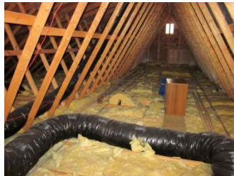
Uneven/ineffective attic insulation found
