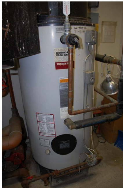
Domestic Hot Water
