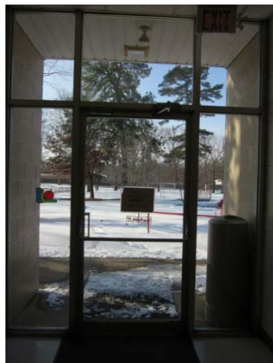
Missing/worn weather-stripping
