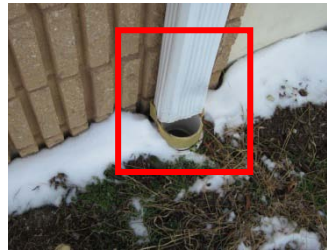
Missing connection between gutter and drain
