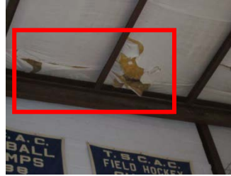
Damaged acoustic ceiling insulation in most areas
