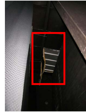
Sagging acoustic ceiling insulation in most areas
