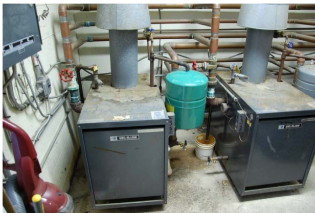
Weil McLain boilers, no signs of rusting yet
