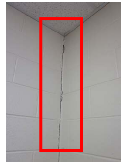
Cracked/deteriorated mortar joints
