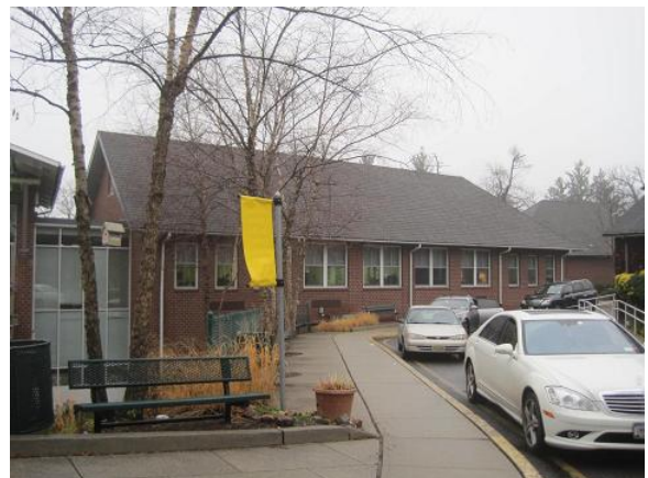
Image 2 exterior façade and bridge
