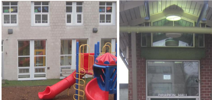
Image 32 & 33 Typical wall mounted and ceiling mounted halogen fixtures
