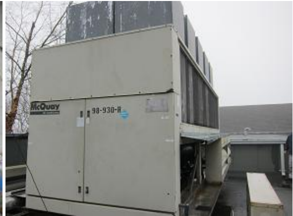
Image 20 Air cooled chiller
