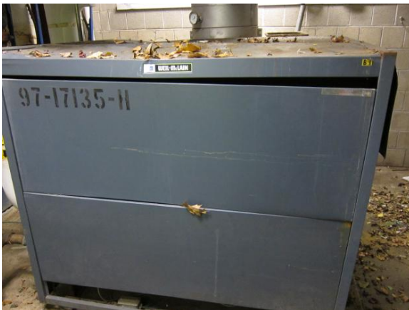
Image 16 (above) Weil-McLain boiler
