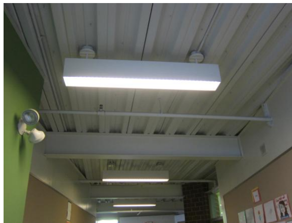
Image 29 Typical Corridor T8 lighting
