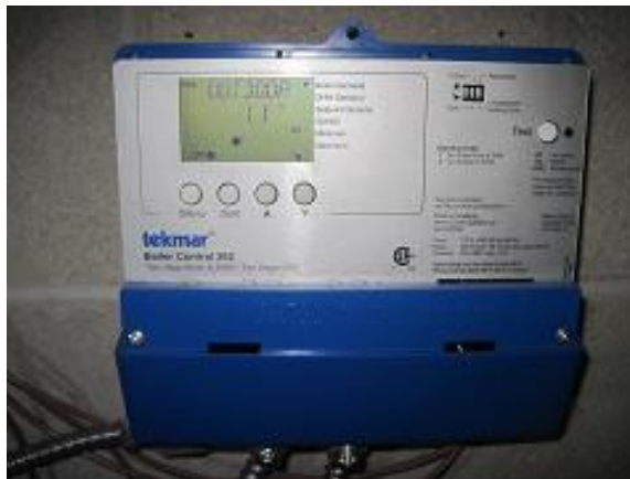
Image 27 Tekmar Boiler Controller
