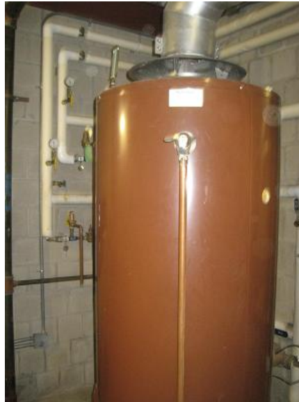
Image 26 A.O. Smith gas-fired DHW boiler
