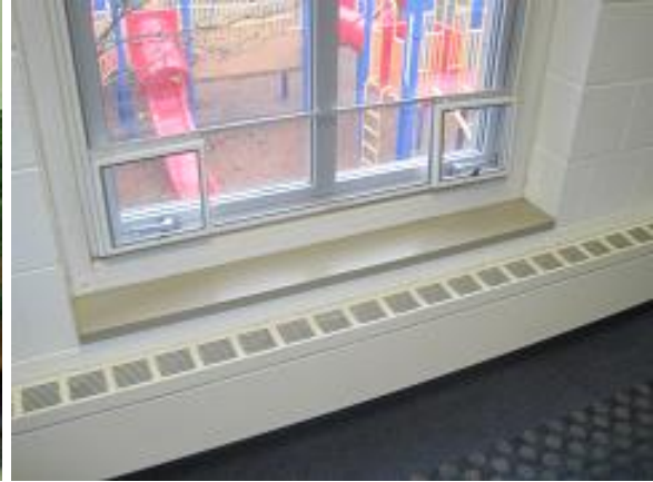
Image 22 Hallway Fin-Tube Radiators
