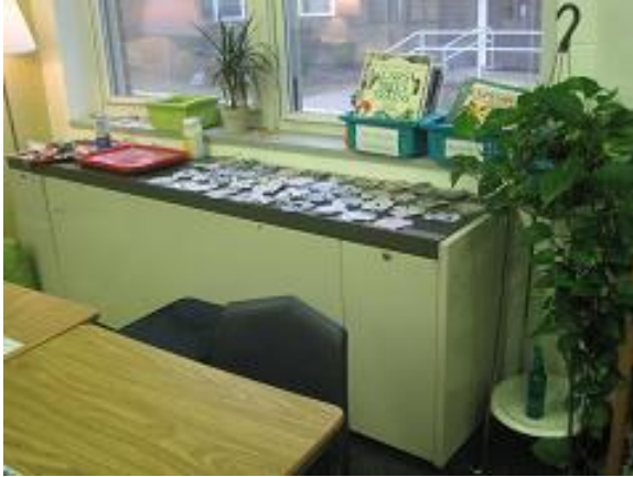
Image 21 Thru-Wall Unit Ventilator
