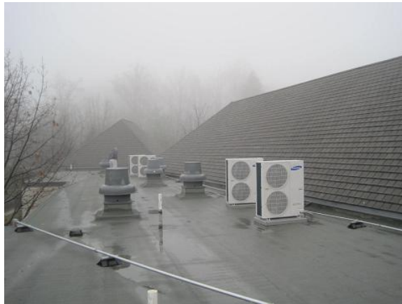
Image 10 Toilet exhaust fans and DX Units
