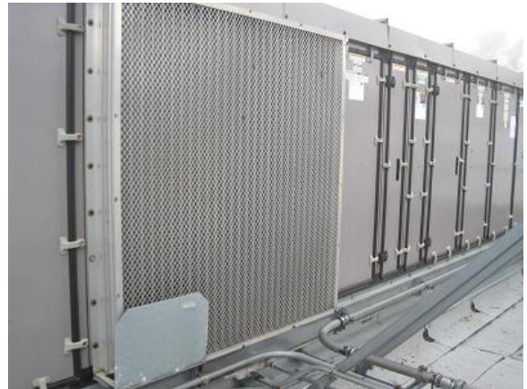
Image 10 Rooftop air handling unit serve the Hajjar Auditorium
