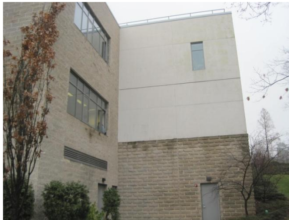
Image 5 Discoloration on split face CMU indicates moisture in the wall cavity
