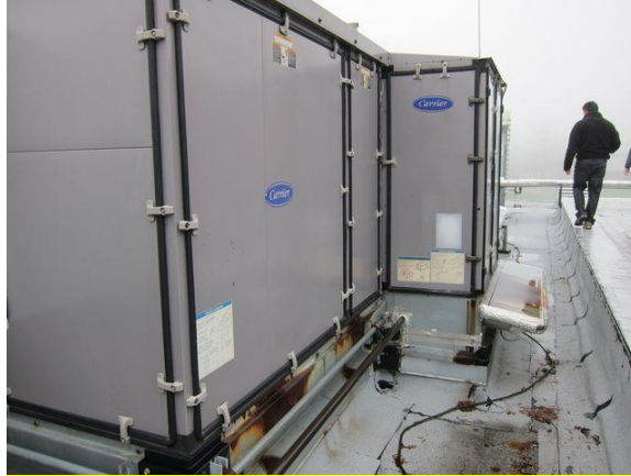
Image 6 The roof section above shows debris collecting on the surface. This can lead to clogged roof drains and roof leaks.
