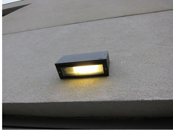
Image 13 Exterior CFL fixture
