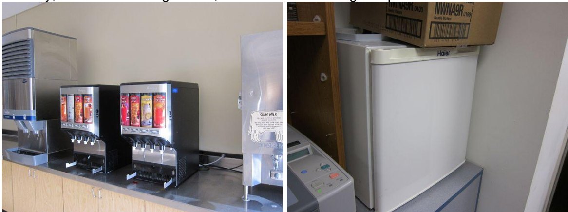
Image 14 Typical “plug load” appliances found in the cafeteria and office spaces
