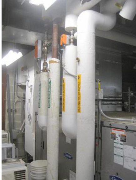
Image 9 Chilled water pipes lack proper insulation near the three-way valve
