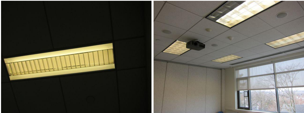
Image 12 Typical T8 fixtures
