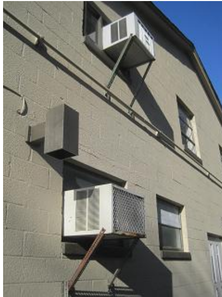
Image 7: AC units installed in winter
