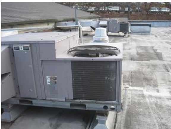
Image 13: packaged units serving small gymnasium
