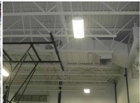
Image 14: Unit ventilator with reheat serving large gymnasium
