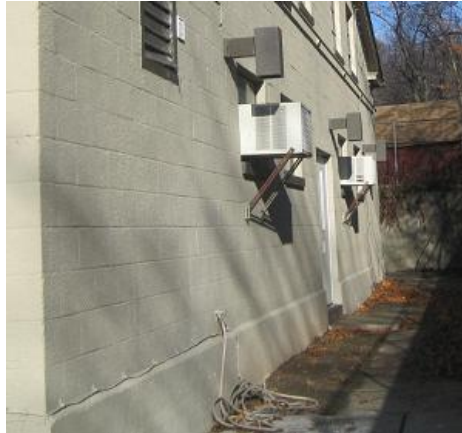
Image 22 Exterior Halogen Lights
