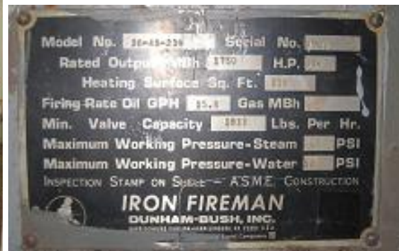
Image 11: Boiler Nameplate Information
