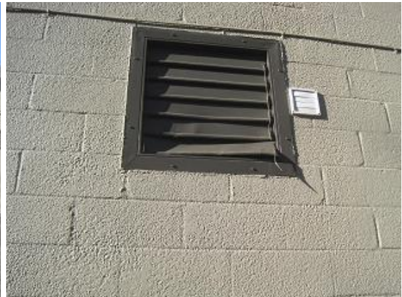
Image 4: Dampers bent, may no longer function.
