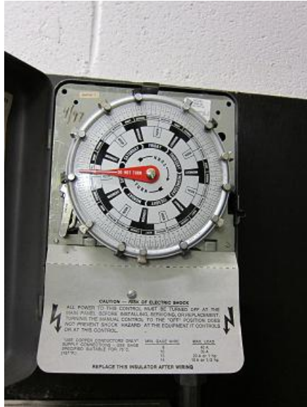
Image 15 Unit Ventilator Timers
