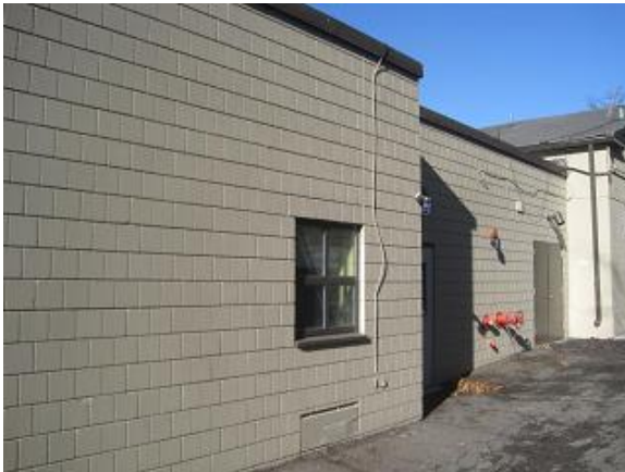
Image 3: CMU exterior appears in good condition.
