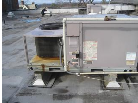
Image 6 roof top units (RTUs)
