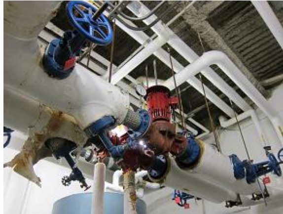
Image 12: Gymnasium HHW Pumps
