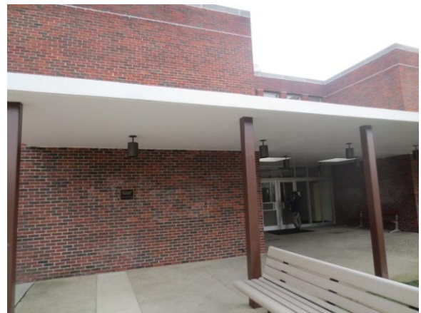
Image 2 Main entryway and typical wall profile
