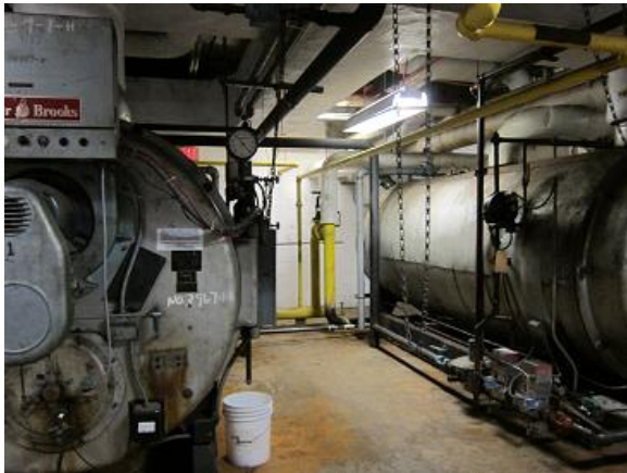
Image 16 Cleaver Brooks boilers
