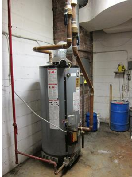
Image 22 Rheem gas-fired DHW boiler
