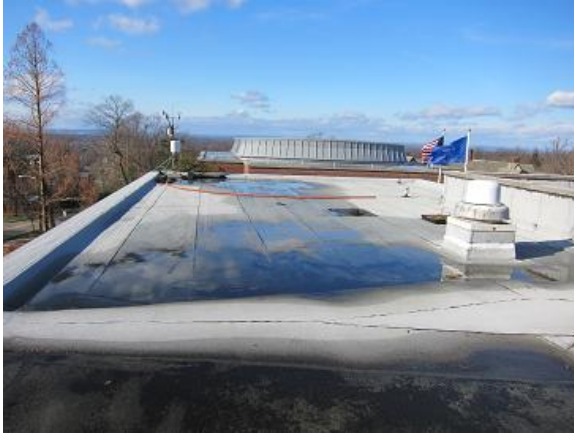
Image 7 Pooling on roof
