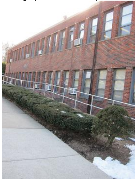
Image 11 Heat escaping through the non-insulated window frames and between AC unit and frame.
