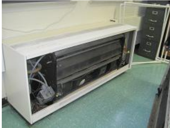
Image 20 Wall Unit Ventilator
