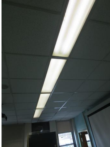
Image 23 Typical Light Fixtures
