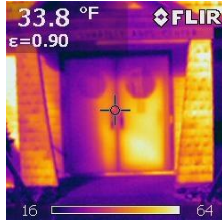
Image 10 Infrared image of front entrance
