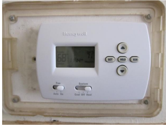
Image 26: Wall mounted thermostat for mini split DX
