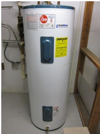
Image 27: DHW Heater tank
