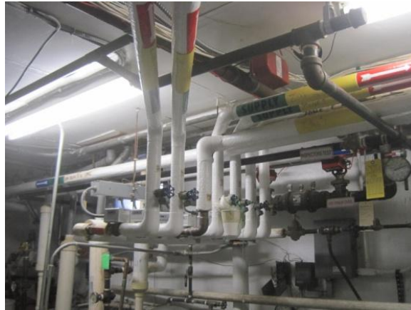
Image 14 Zone control valves for heating loop
