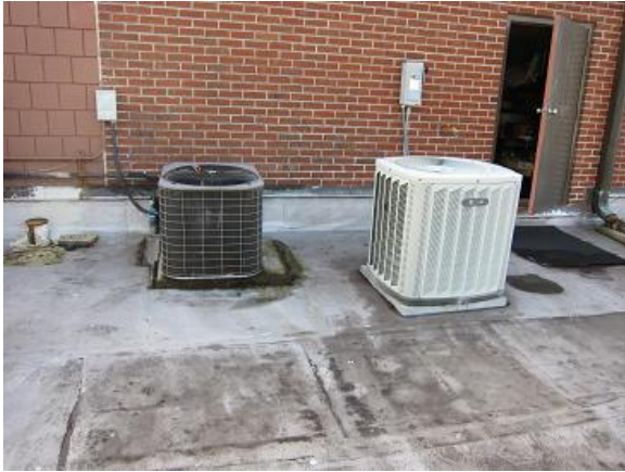
Image 14 Ductless Split Units
