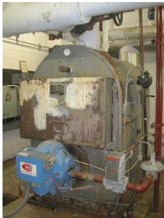
Image 11: Dunham-Busch Hot Water Boiler
