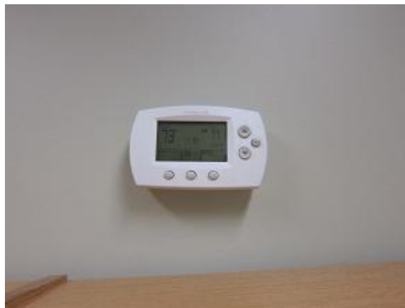
Image 16 Room Thermostat controlling RTU
