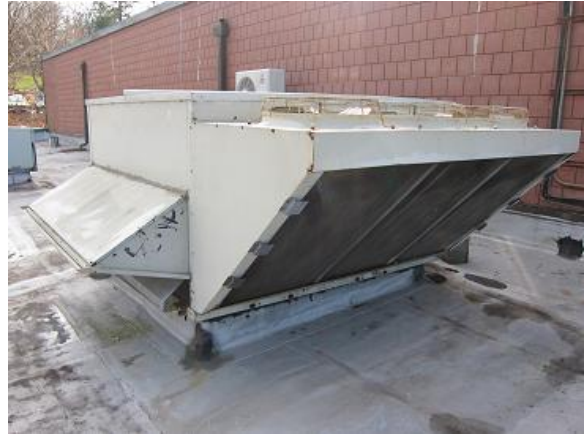
Image 15 RTU-1 serving main area
