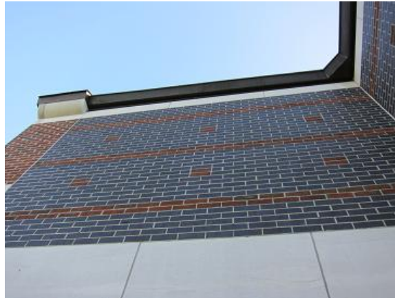
Image 3 Brick facing on exterior walls
