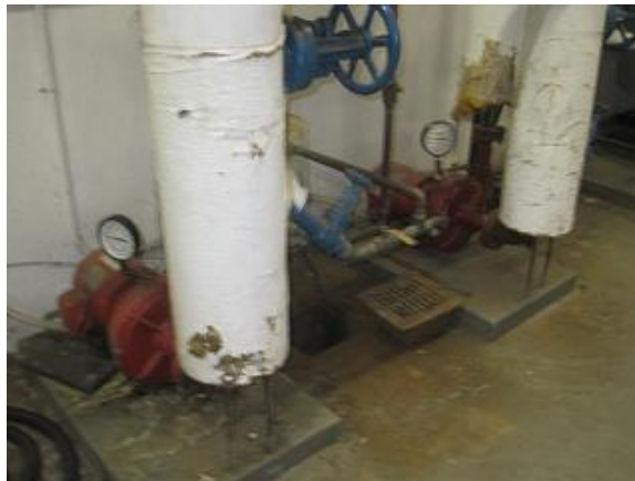
Image 13: Library HHW Pumps
