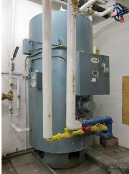
Image 17 Electric Immersion water heater
