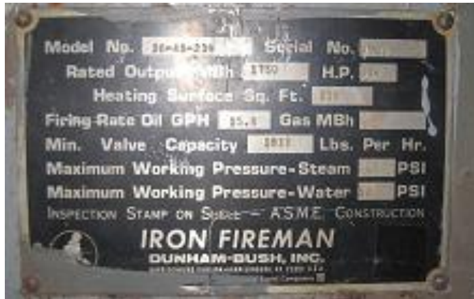
Image 12: Boiler Nameplate Information
