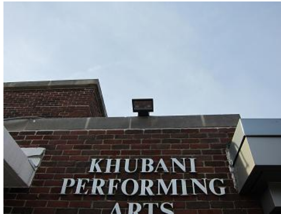
Image 17 Exterior Halogen lights
