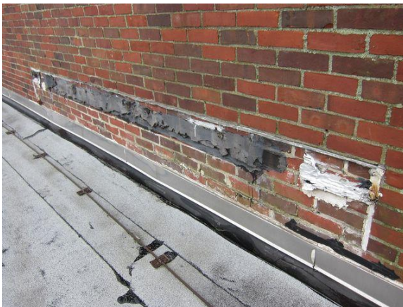
Image 4 deficiencies in exterior wall
