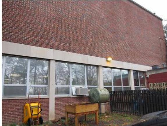
Image 7 Rear windows and window AC
