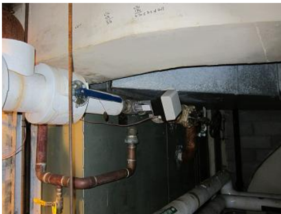
Image 12 Air Handling Unit
