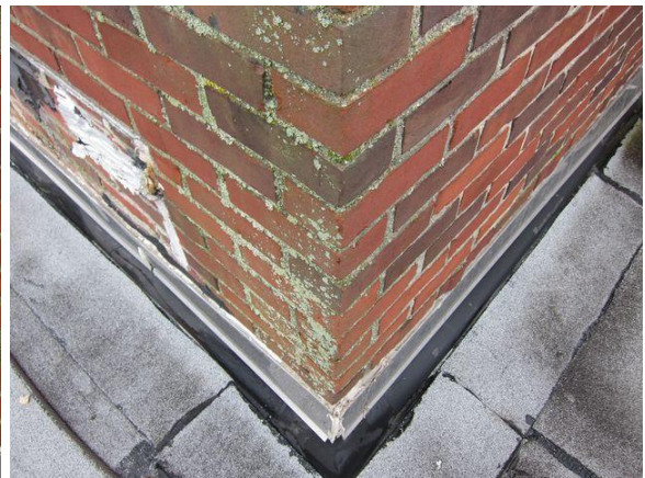
Image 5 cracking and discoloration in bricks and mortar
