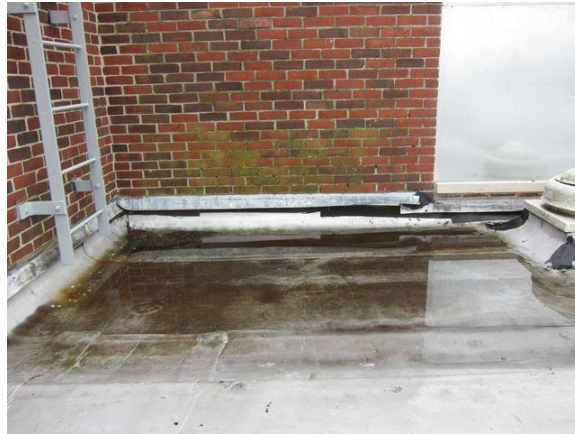
Figure 6 Pooling/standing water above auditorium
