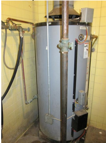
Image 15 Gas-fired DHW heater
