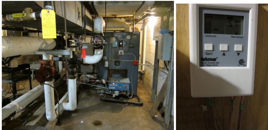
Image 9 Weil McLain boiler and Tekmar controller
