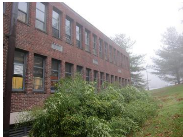
Image 2 rear of building
