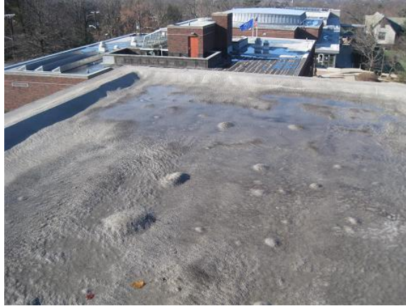
Image 4 bubbling on roof
