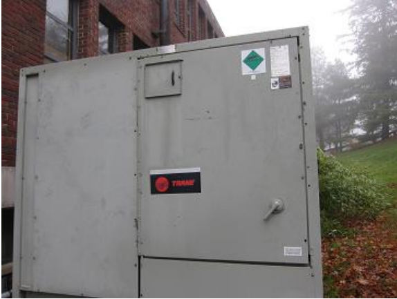
Image 10 air cooled chiller
