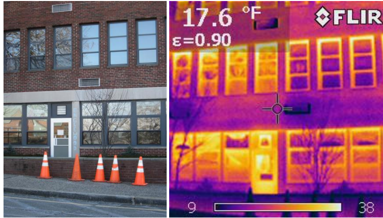
Image 7 Infrared image of Umpleby Hall windows
