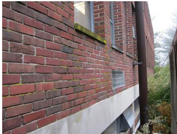
Image 3 typical brick exterior
