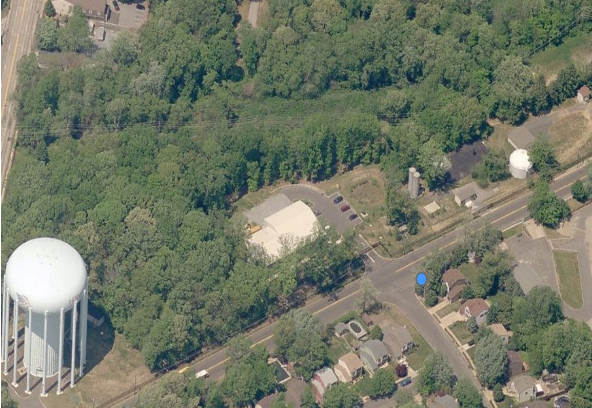
Figure 1: Park Avenue Water Treatment Plant
